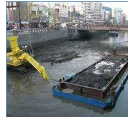
Dredged soil from rivers and harbors
