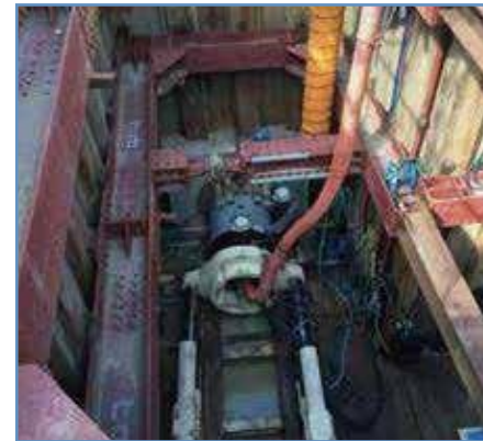
Excess mud water generated by propulsion and shield tunneling
