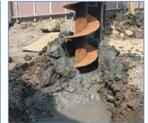
Polluted sludge generated by ground improvement
